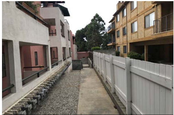
#10 NORTH PROPERTY LINE FENCE
