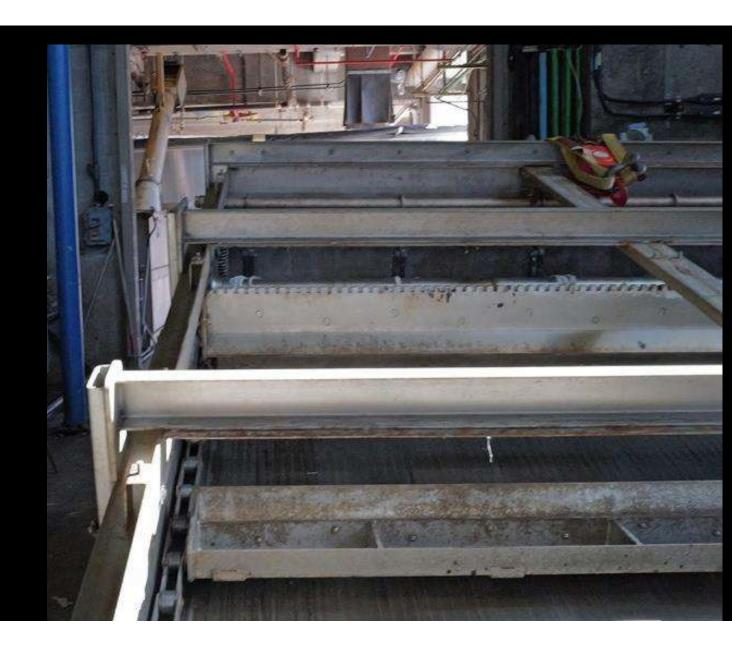
This is one of our tour group inspecting the screenings flume. In the back ground, on the wall you can see one of the new video cameras (white band in the middle). This is a critical point to transport screening out of the building and a failure of the type in 2021 could be seen here.
