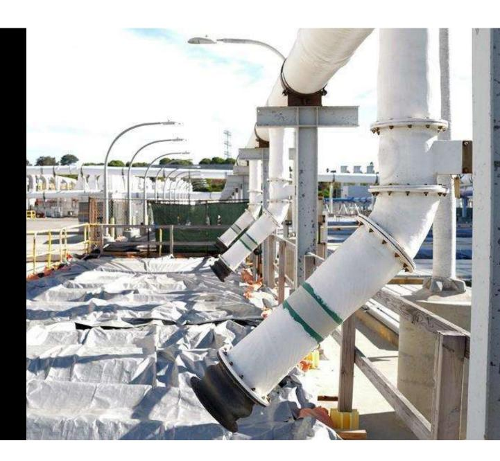
This slide shows the covers for the third and fourth batteries of primary clarifiers. The green hill on the right is the plant's border with the City of El Segundo. The removable aluminum covers lie flat on the deck. They are always removable at treatment plants to allow maintenance. The white pipes are to transport foul air.
