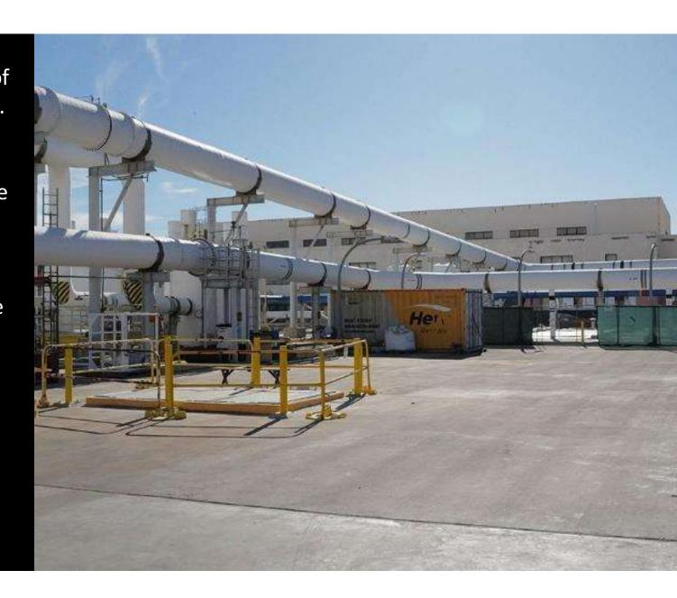
Here is a detail of the odorous gas piping. It extends around the plant. Buildings that have odor producing processes are always sealed up and connected to odor control piping.
