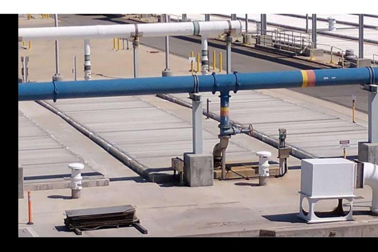
The odorous gases are transported to odor control towers. Here the gas is contacted with water containing chemicals that reactor with the odors to remove them. There are also towers that use activated carbon. Newer towers are using biomass to oxidize the odors.
