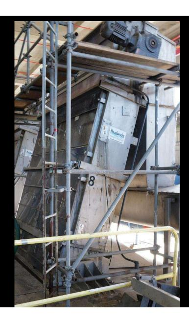
This slide shows the back of the bar screens. They are covered to reduce odors. During the worst of the flood, screenings covered the floor you see and it was approximately 2 ft underwater.
