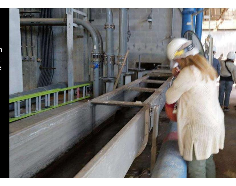
This slide shows one area of the primary clarifier covers. They are partially covered with removable panels and partially with fixed concrete covers. Primary clarifiers always have movable parts which require routine maintenance and therefore access. The primary clarifiers are operated under a partial vacuum so that odorous gases can be sucked through the large pipes to an odor control facility.
