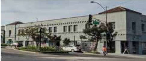
105 W. Grand Avenue is prominently situated at the corner of Grand Avenue and Main Street and is an example of an existing mixed-use commercial building
