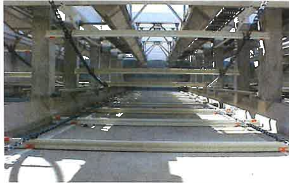
REPLACE SLUDGE HANDLING EQUIPMENT
