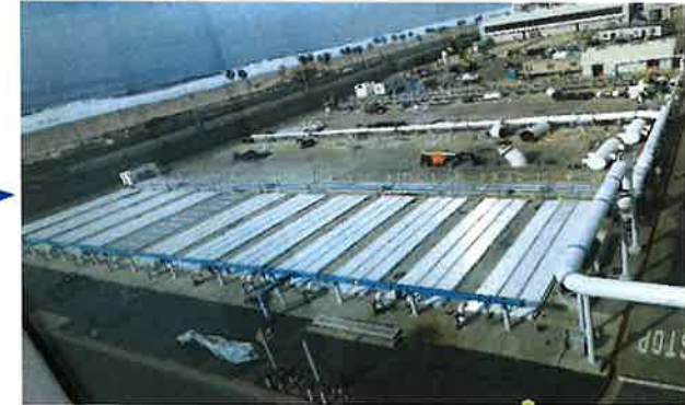
REPLACE TANK COVERS
