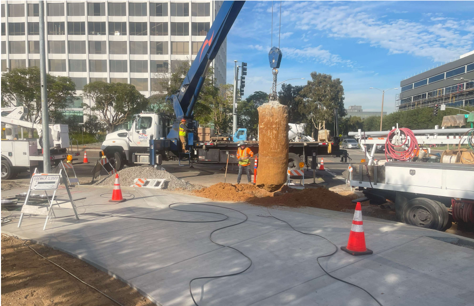
Removal of existing concrete foundation for the traffic signal pole.
