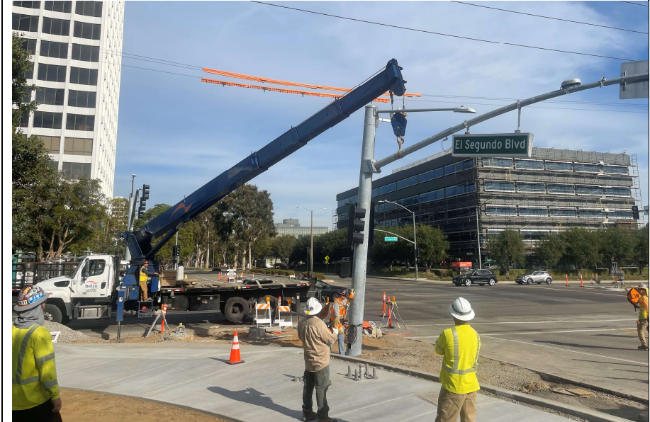
Relocation of traffic signal pole at El Segundo Blvd and Continental Blvd.
