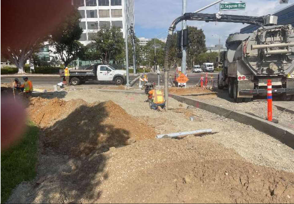
Removal of existing concrete foundation for the traffic signal pole.
