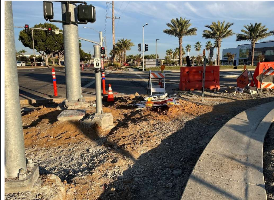
Traffic signal poles need to be adjusted to behind the new curb.
