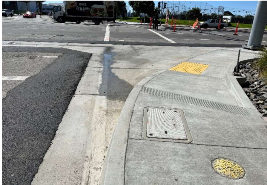
Drainage repairs, ADA improvements, pedestrian push button upgrades.
