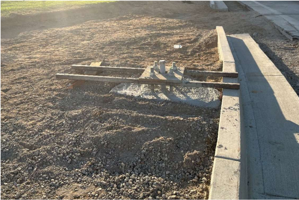
Setting new concrete foundations for traffic signal poles.
