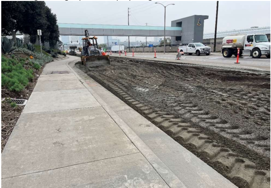
Removing existing asphalt and preparing subbase.
