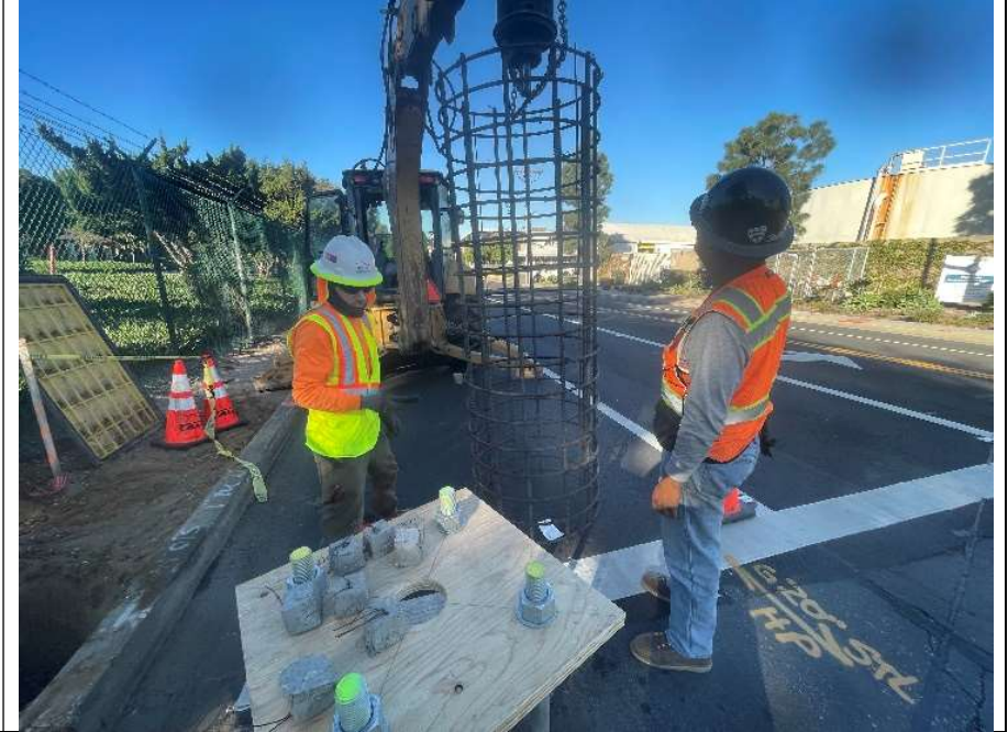
Relocation of traffic signal pole at El Segundo Blvd and Continental Blvd.
