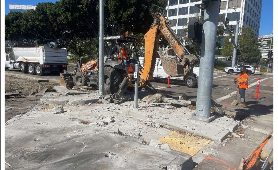
Traffic signal poles need to be adjusted to behind the new curb.
